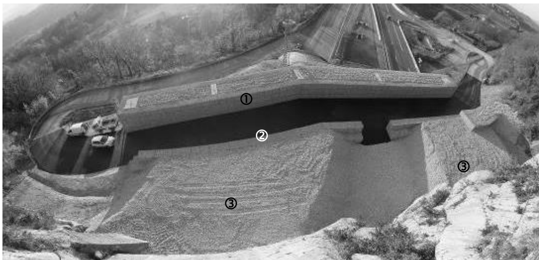
Figure 6: Sights of the finished embankment
