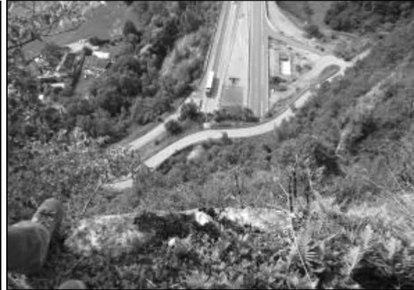
Figure 2: Sight of the highway from the top of the cliff
